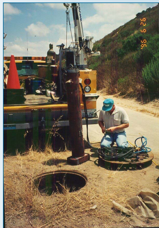
DEPLOYMENT IN SEWERS FOR TOMOGRAPHY
