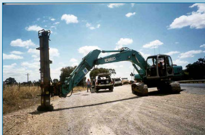
CHURCHILL DROP SOURCE IN USE ATTACHED TO 22 TONNE EXCAVATOR
