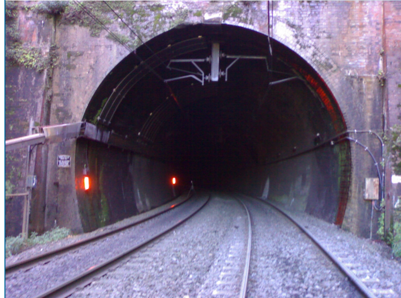
ENTRANCE TO A BRICK LINED RAIL TUNNEL
