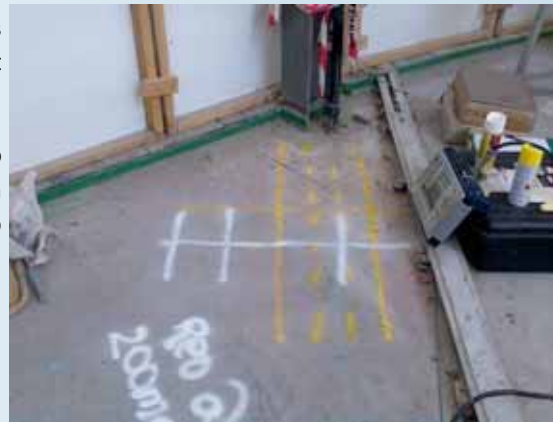
INTRA-SLAB STEEL MARKED ON SITE DURING SURVEY
