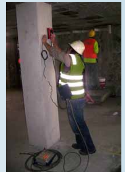
1.5GHZ ANTENNA USED TO SCAN CONCRETE COLUMNS
