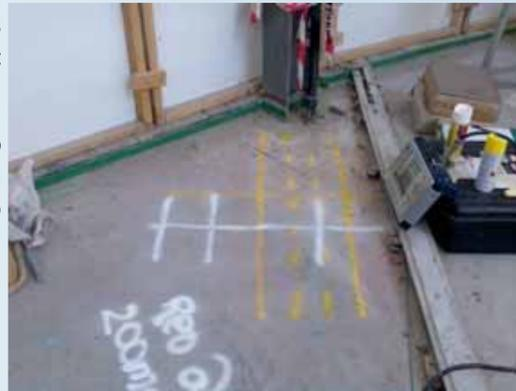
INTRA-SLAB STEEL MARKED ON SITE DURING SURVEY
