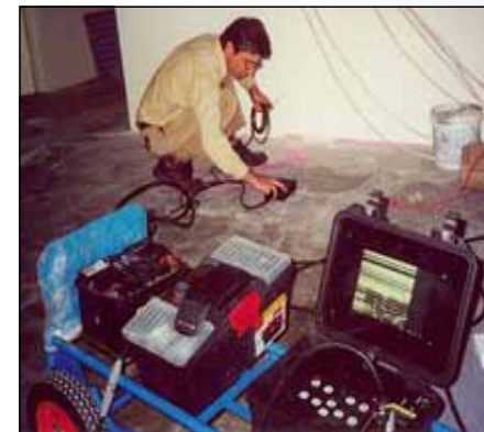
USING 1.2GHZ ANTENNA FOR TENDON DUCT LOCATION
