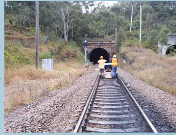
GPR data collection along a section of rail track.
