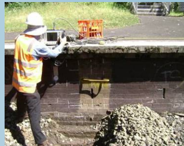
GPR investigation to determine wall thicknesses at a station platform.
