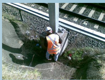
Impact-echo investigation to determine pile depths of overhead structures
