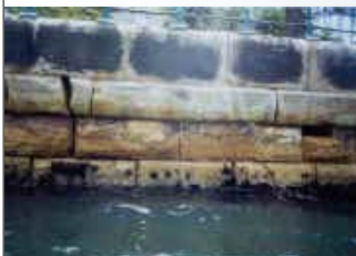
VERTICAL CRACKING IN WALL ON CURVED EASTERN SECTION, INDICATING PAST OUTWARD MEVEMENT OF THE WALL
