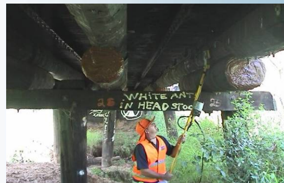
Radar profiling timber girders at Redbank bridge QLD.
